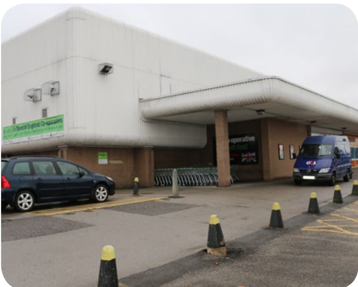
View of the store from the site entrance
