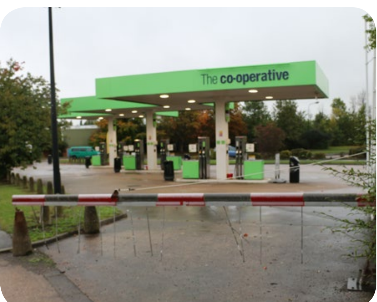
View of the petrol filling station from the south of the site
